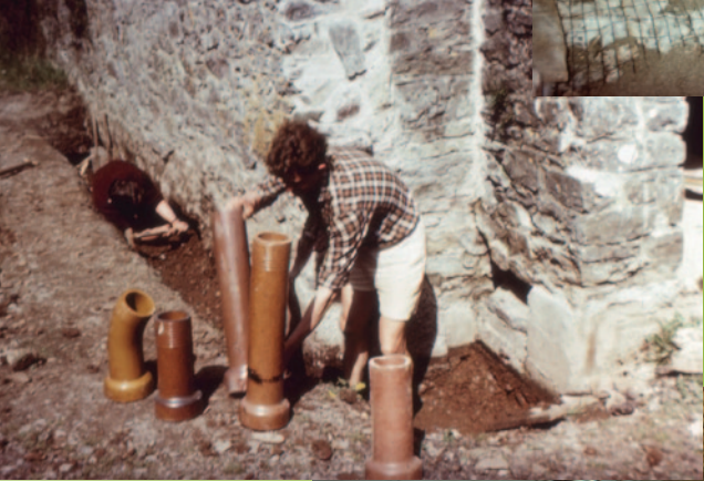
Left: Bill Maxwell working on the drainage
