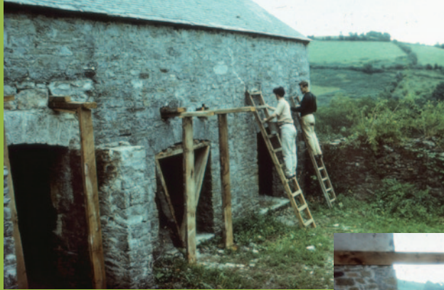
Above and right: Securing the structure of the barn and pouring concrete for the floor, 1963
