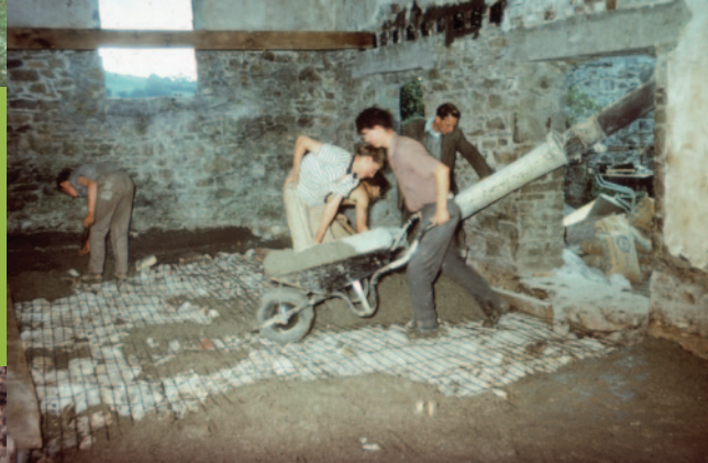
Above and right: Securing the structure of the barn and pouring concrete for the floor, 1963
